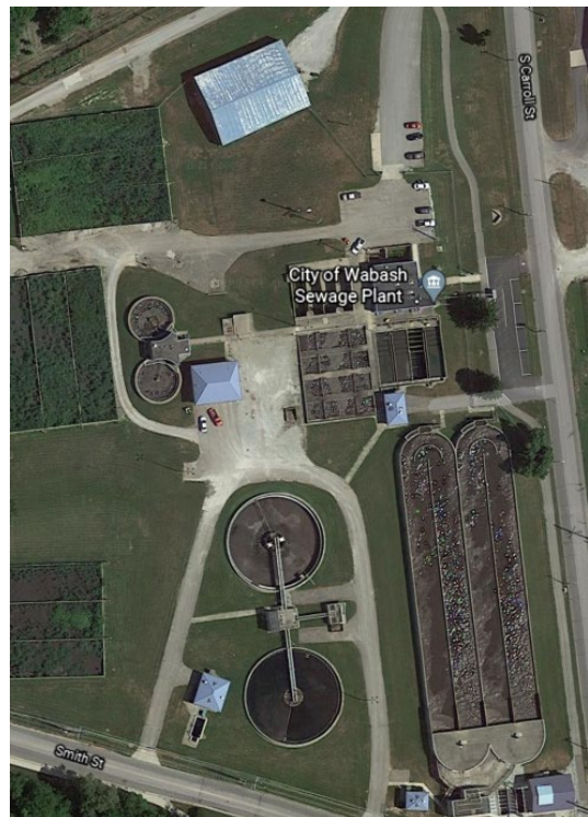
Figure 4-6: City of Wabash Sewage Plant
