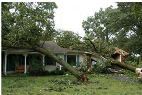
Figure 3-17 Home Damaged During Windstorm
