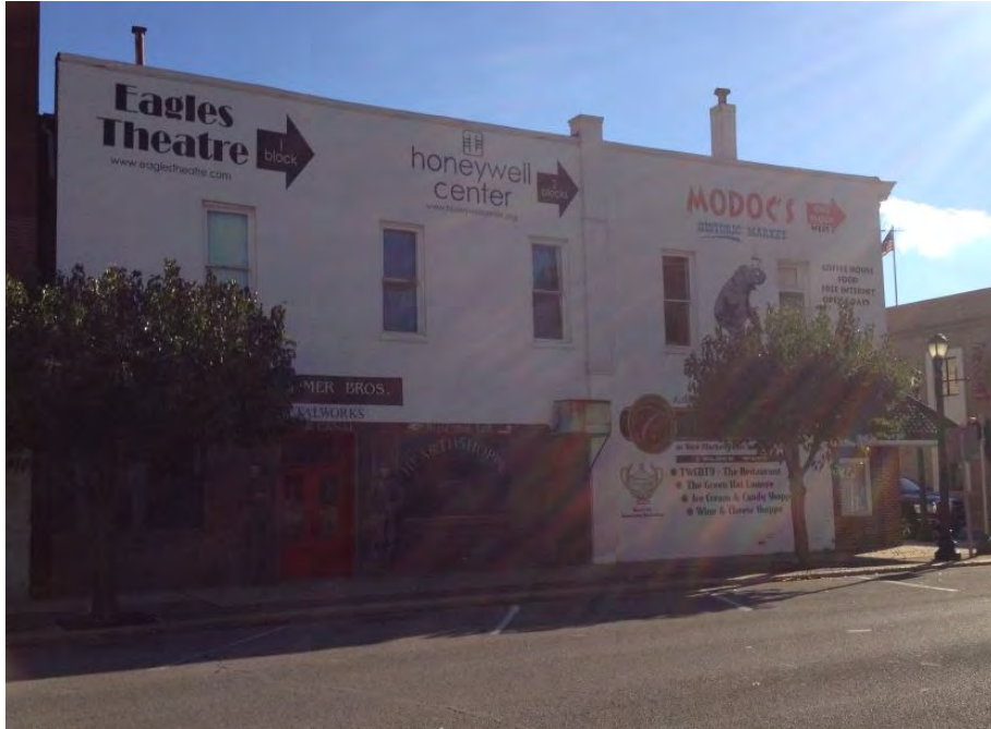
Building adjacent to the west
