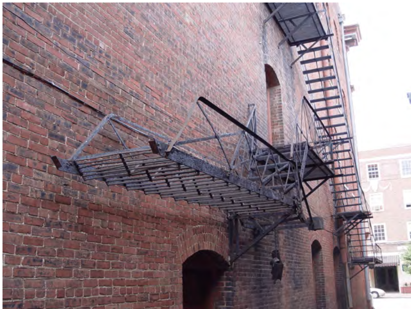
West Fire Escapes
