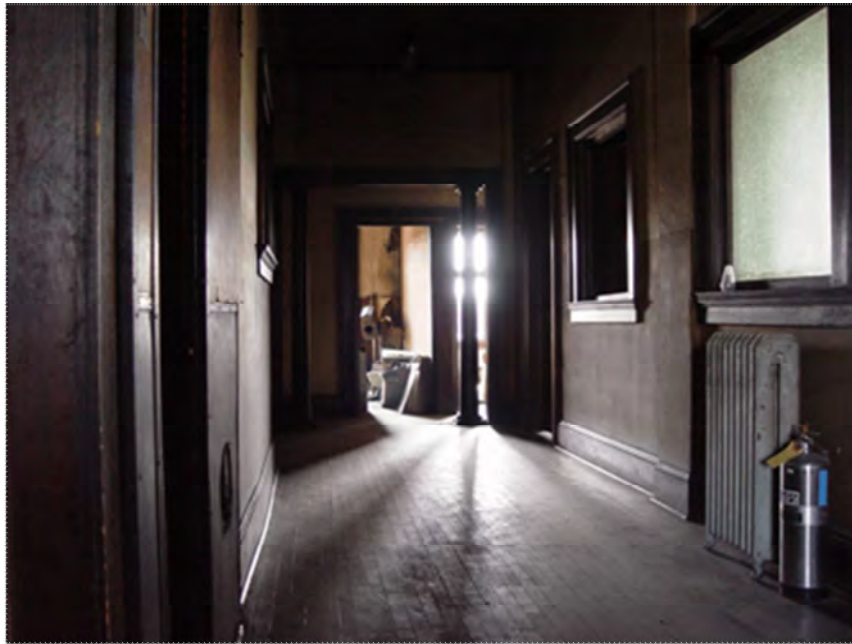
Fourth Floor Hallway
