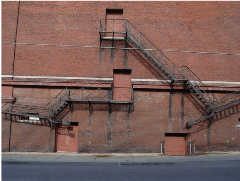
East Fire Escapes
