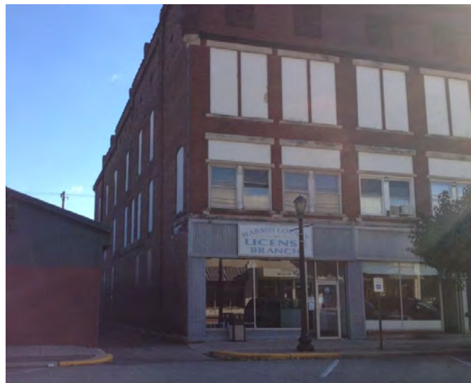
Looking at the southeast side of the building.
