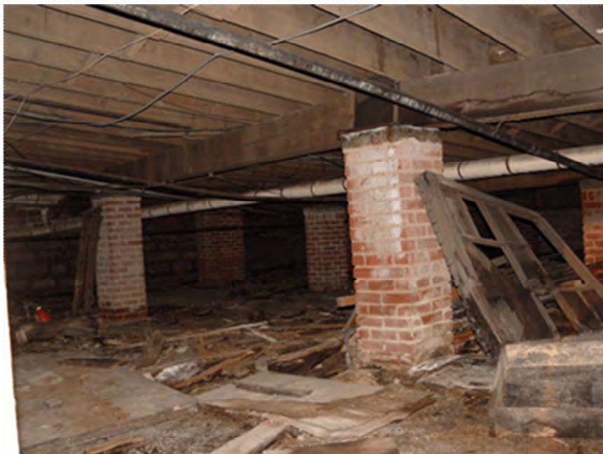
Sloped Wood Structure under Main Floor
